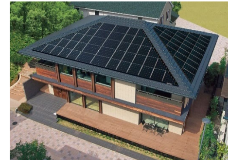
<Image of solar power generation system installed>
