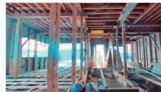
Structural frame being reused
