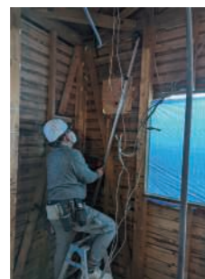
Seismic reinforcement work
