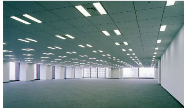
"Grid-system ceiling" to respond flexibly to a change in office layout
