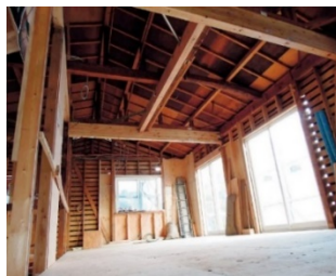
Interior stripped down to its main frame
