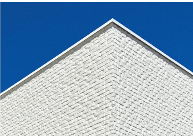
Oxidizes harmful pollutants such as NOX (nitrogen oxides) found in vehicles' exhaust gas into harmless ions, which are washed away with rain. Its air purification capacity is 165 m<sup>2</sup> (approximately one house), equivalent to 12 poplar trees.
