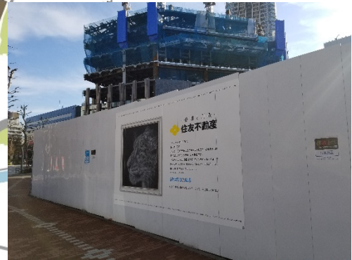
Displayed artwork and the building under construction
