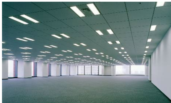
"Grid-system ceiling" to respond flexibly to a change in office layout
