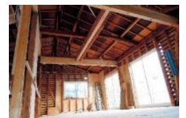
Interior stripped down to its main structural elements
