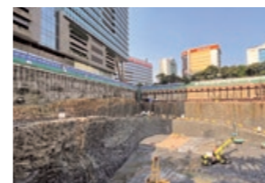
Project 1 in BKC (underground excavation is underway)
