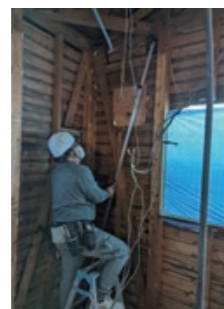
Seismic reinforcement work
