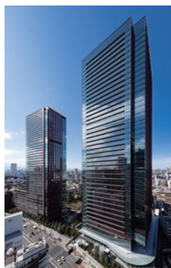
Sumitomo Fudosan Tokyo Mita Garden Tower (Completion: Feb 2023) Shinjuku Ward, Tokyo No. of floors: 42 above / 4 below ground Gross floor area: 196,214 m 2
